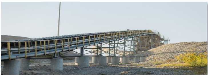
Six data center projects in the Kansas City Region are currently supplied by Martin Marietta's differentiated Central Division
